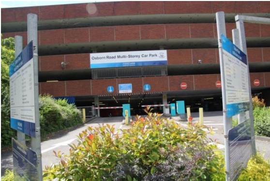
Osborn Road Multi-Storey Car Park
